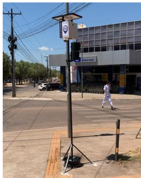
Figure 5. Image acquisition system installed and operating.
