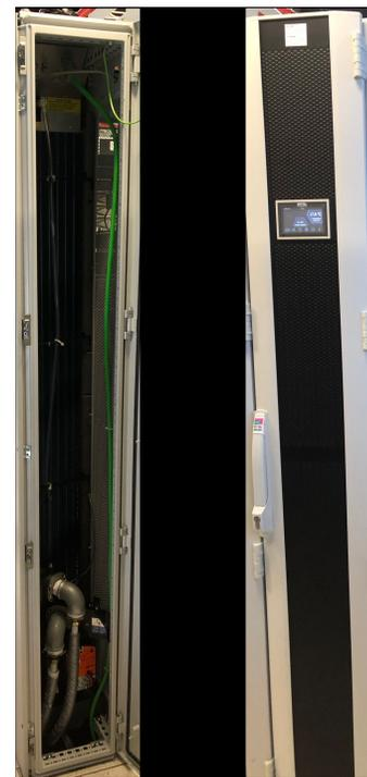
Fig. 6. Liquid Cooling Package - LCP
