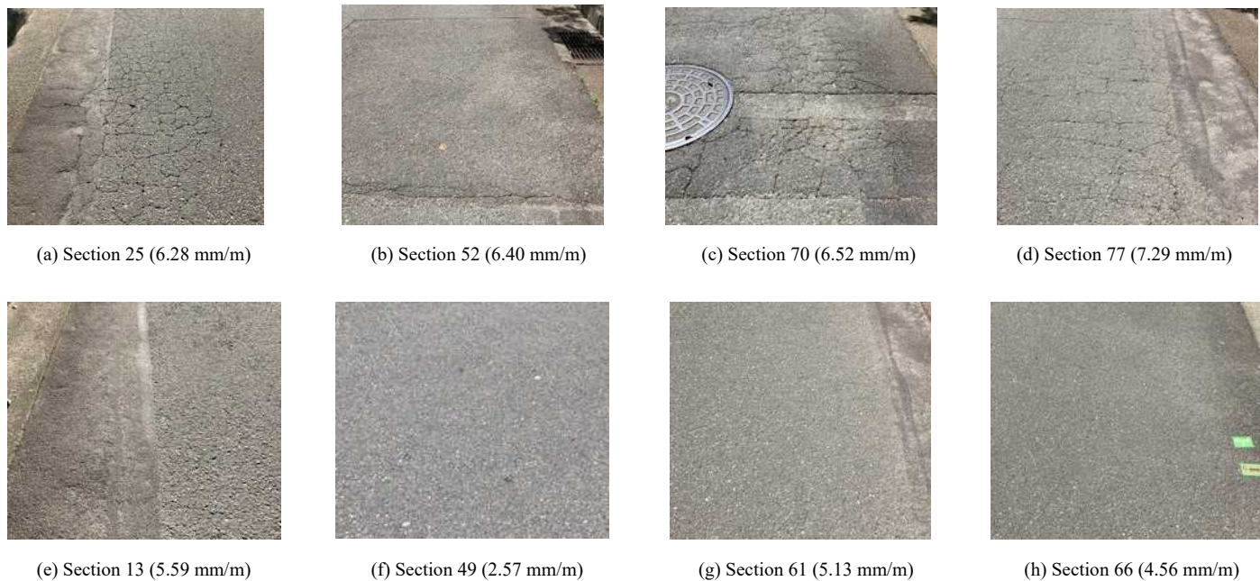
Figure 17. Photo of road surfaces in eight sections. Numerals in brackets indicate the estimated IRI values. The IRI level of (a)–(d) is high (yellow circle in Figure 16), and that of (e)–(h) is low (white and light blue circles in Figure 16).
