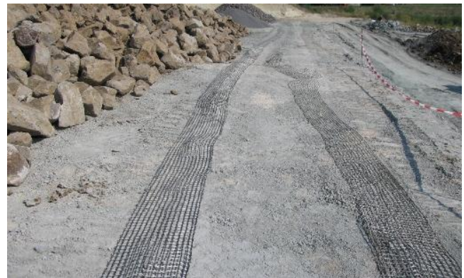
Figure 8: Geogrid with integrated fiber optical sensors.
