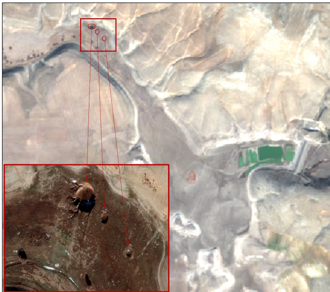
Figure 7. Images of the sinkholes formed in the May Dam (Imagery sources: Google Earth and Copernicus Sentinel data processed by ESA).
