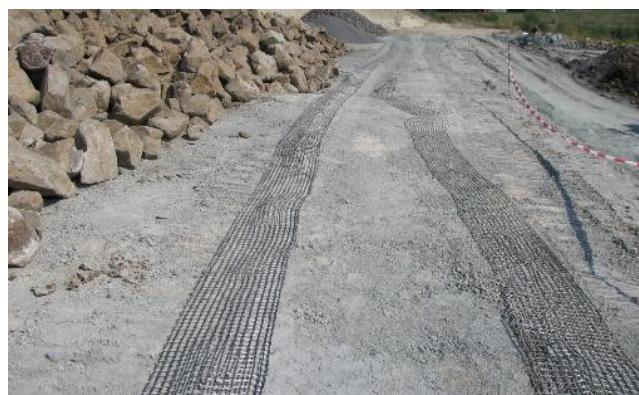
Figure 8: Geogrid with integrated fiber optical sensors.
