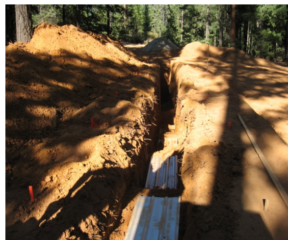
Figure 6. Target GPR imaging objects, tin roofing sheets, were buried at various depths. The experiments provided ground truth GPR data for hardware to software comparison.
