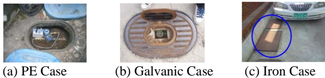
Figure 6. Cover Types for Water Meters
